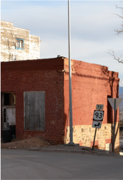
The Amsden brothers lived in this building just down the street from the LCTS central office.
